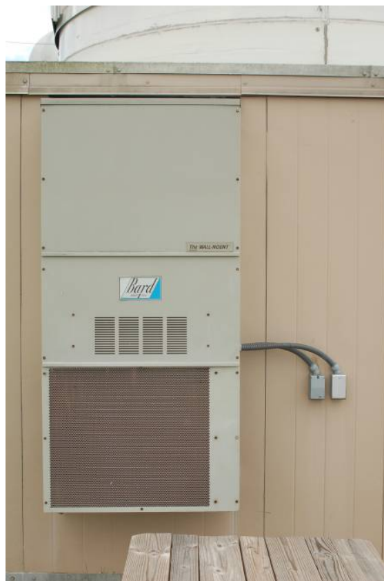
12-3: Wall Mounted HVAC Unit
