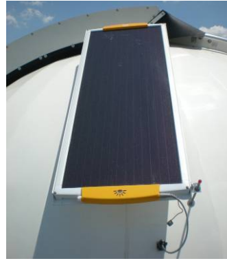
Figure 12-10: Solar Panel to Charge the Battery
