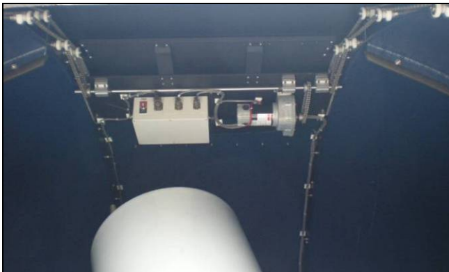
Figure 12-12: Location of Remote Shutter Drive
