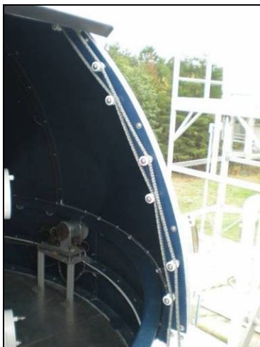
Figure 12-7: Endless loop chain and guide
